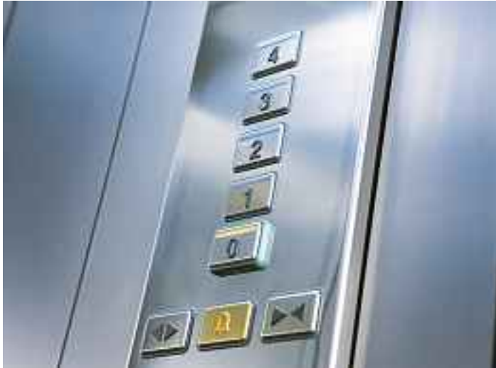
Car operating panel
