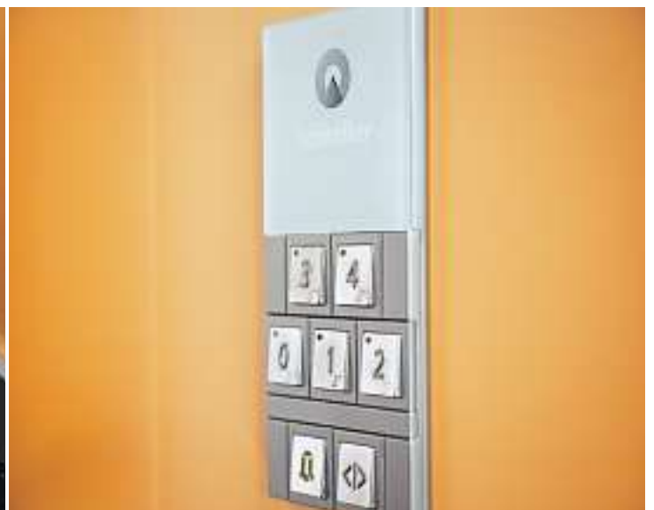
Car operating panel
