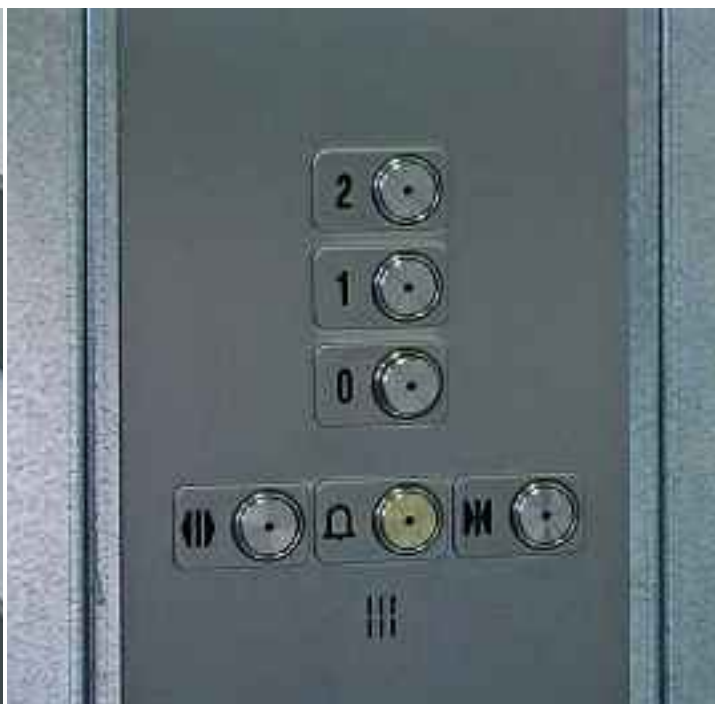
Car control panel of stainless steel, vandal-proof
